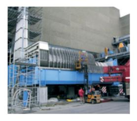
replaced less efficient dewatering equipment. The twin screw press provides for the most cost efficient separation of large quantities of water from materials, which later may be further processed by thermal processes. The twin screw press is applied to sugar beet pulp. In this industry more than 60 percent of the world's factories use the twin screw press.
